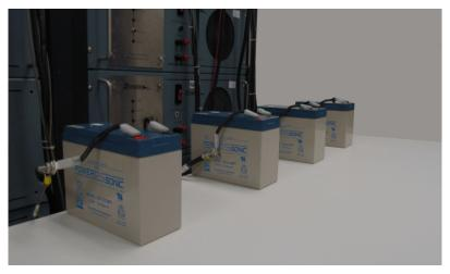
Sulfation is the number one reason you should not store your lead acid battery without charge. Once sulfation of the lead plates has happened, reversing the effects is highly unlikely, so it is essential to look after your batteries from the start.
